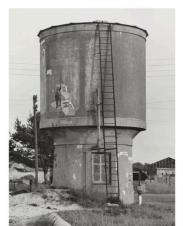
A teleological explanation would cite the purposes or functions of these buildings. They are water towers. So to hold as much water as possible, the upper part is large. And to dispense water by gravity, the building is tall. (Italics are the purposes.)
